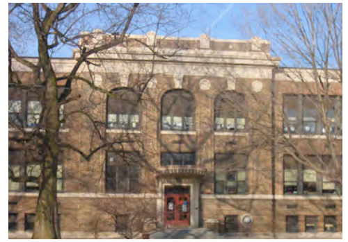
BUTLER ELEMENTARY SCHOOL
