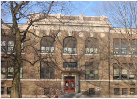
BUTLER ELEMENTARY SCHOOL
