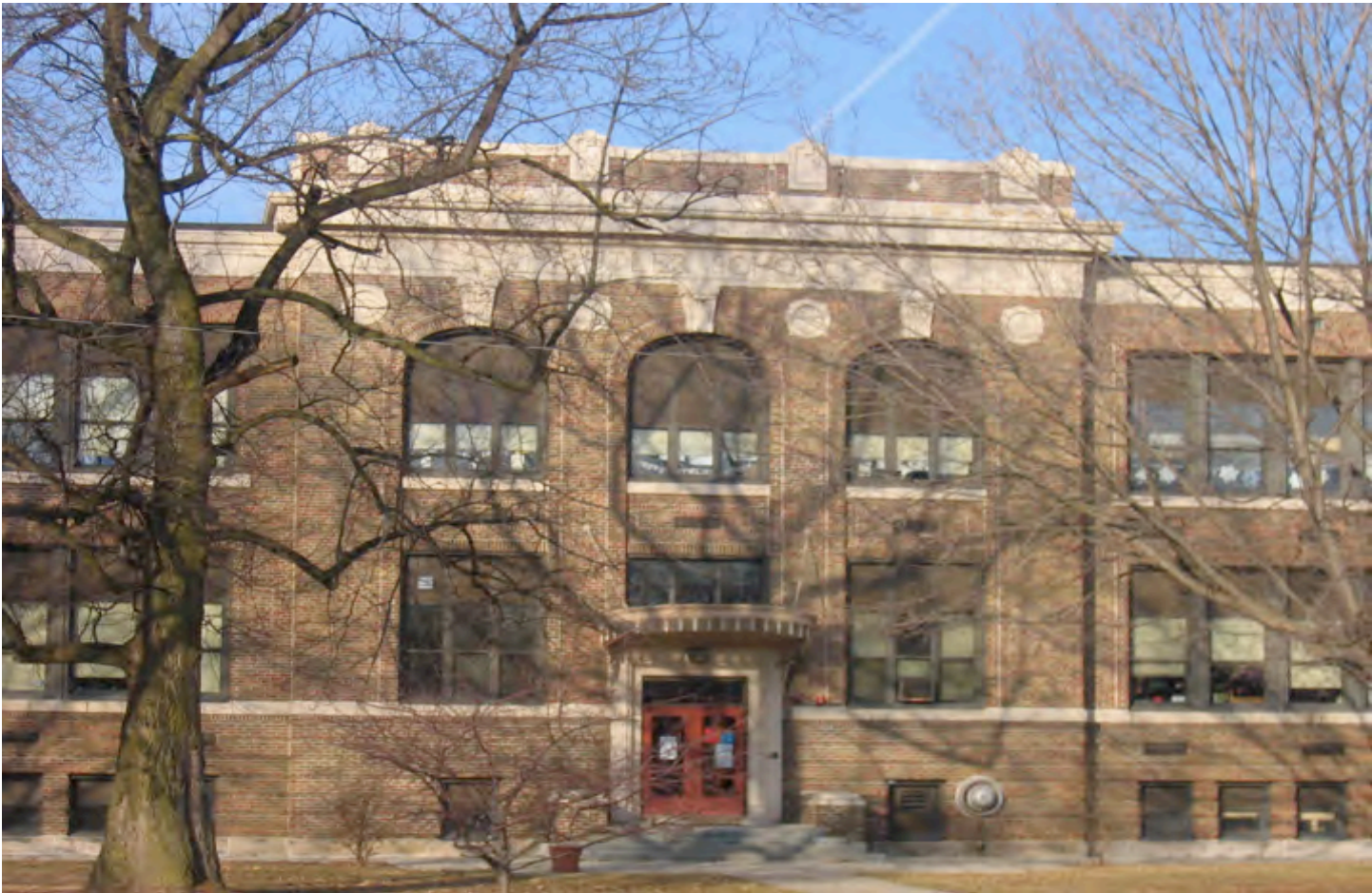
BUTLER ELEMENTARY SCHOOL
