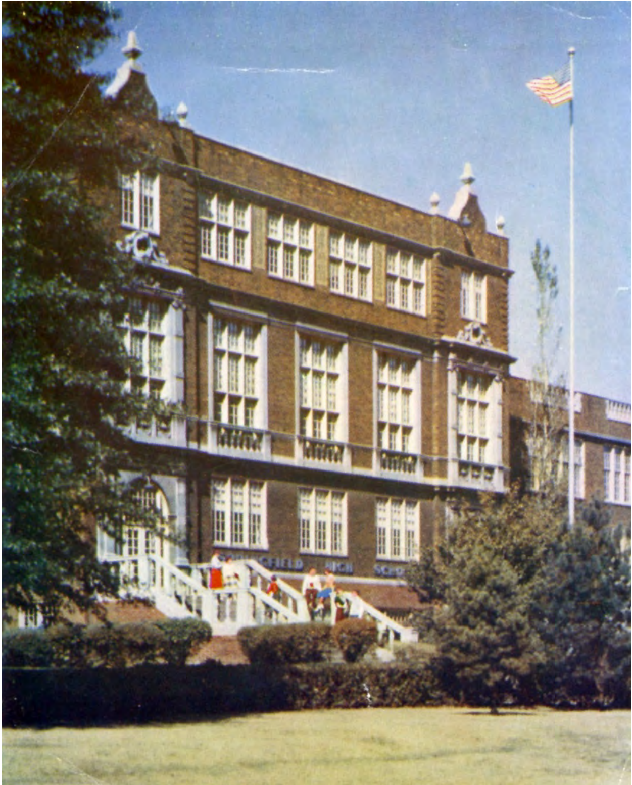
Circa late 1950's illustrating central portion of east elevation with dual entries before significant window modifications and removal of decorative parapet and stone details completed by the start of 1960. Photo courtesy Sangamon Valley Collection Lincoln Library.
